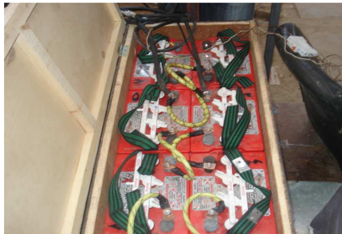
Figure (10) shows the batteries arrangement within a special box.
