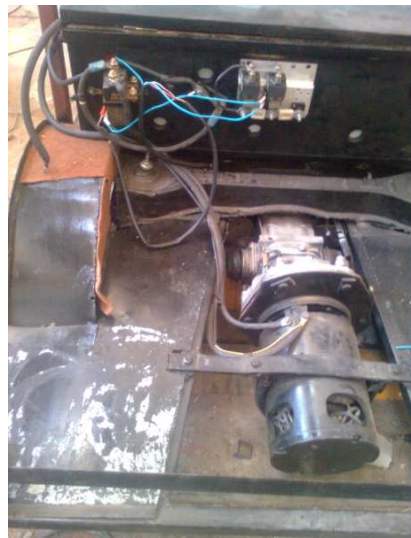
Figure (11) shows the contactors used within the electrical connections.
